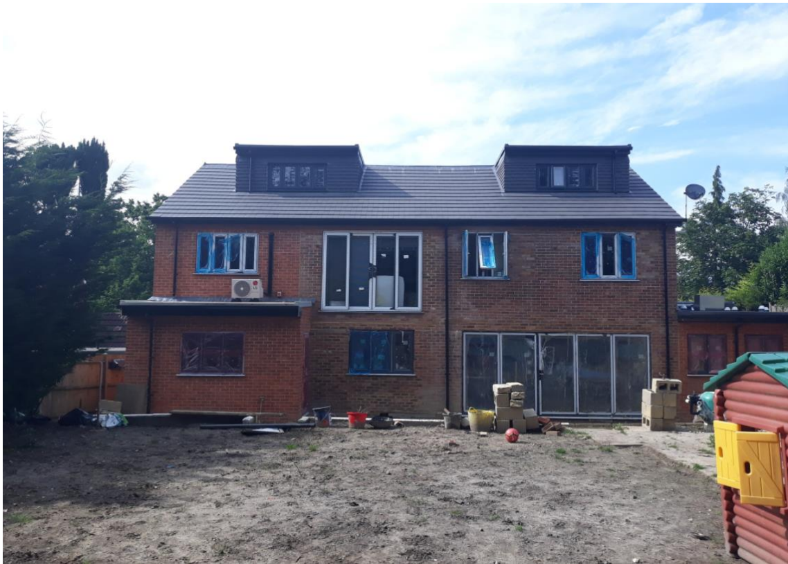
Image of the rear of the application site
